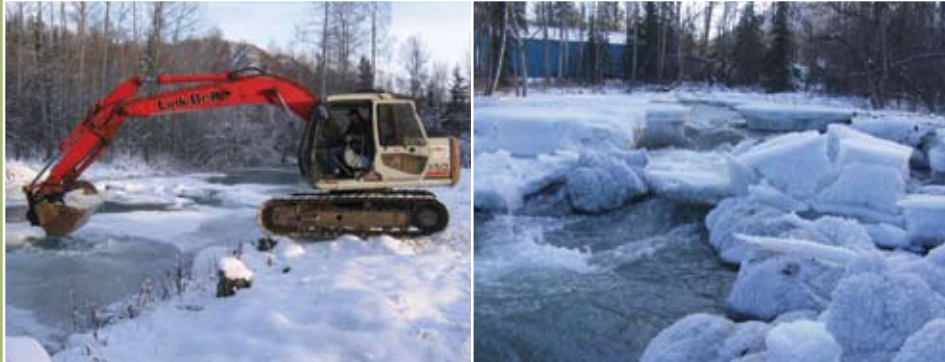
Excavator works to break up ice dams on Peters Creek.
